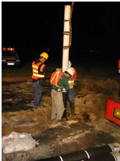
Figure 11 - Construction of vertical vent shaft
