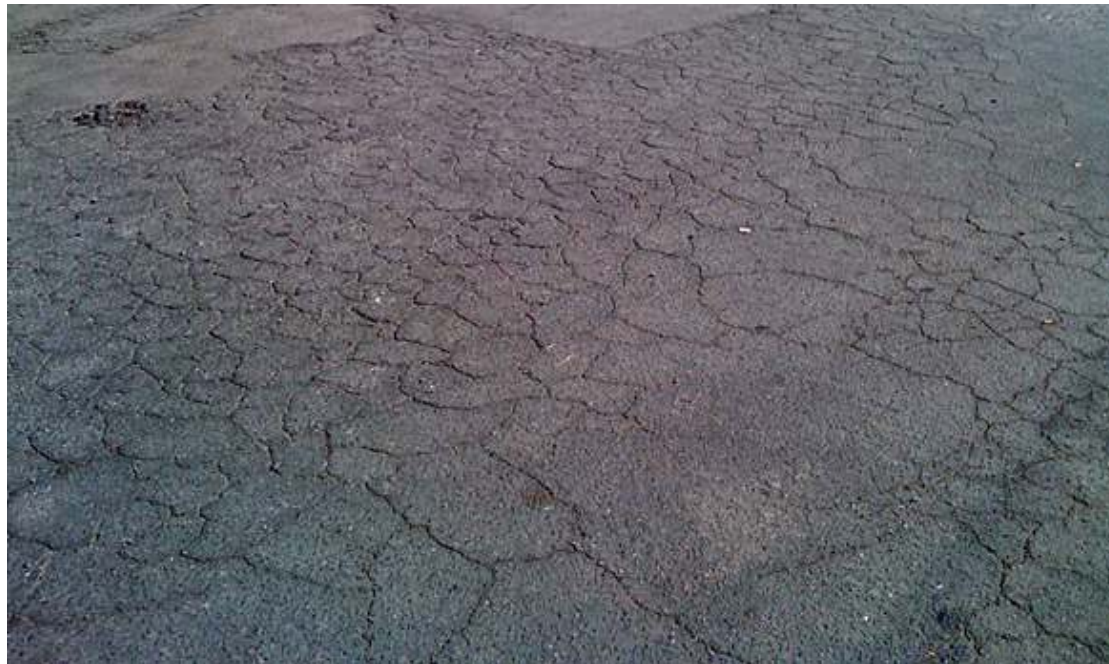
Alligator cracking
